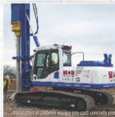
Installation of 200mm square pre-cast concrete pile
