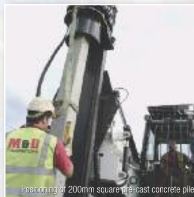
Installation of 200mm square pre-cast concrete pile
