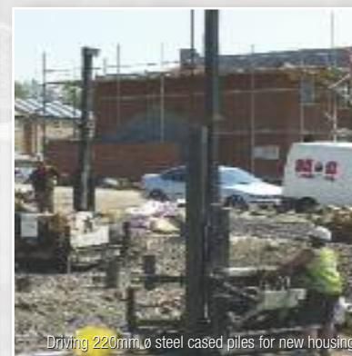
Driving 220mm \emptyset steel cased piles for new housing
